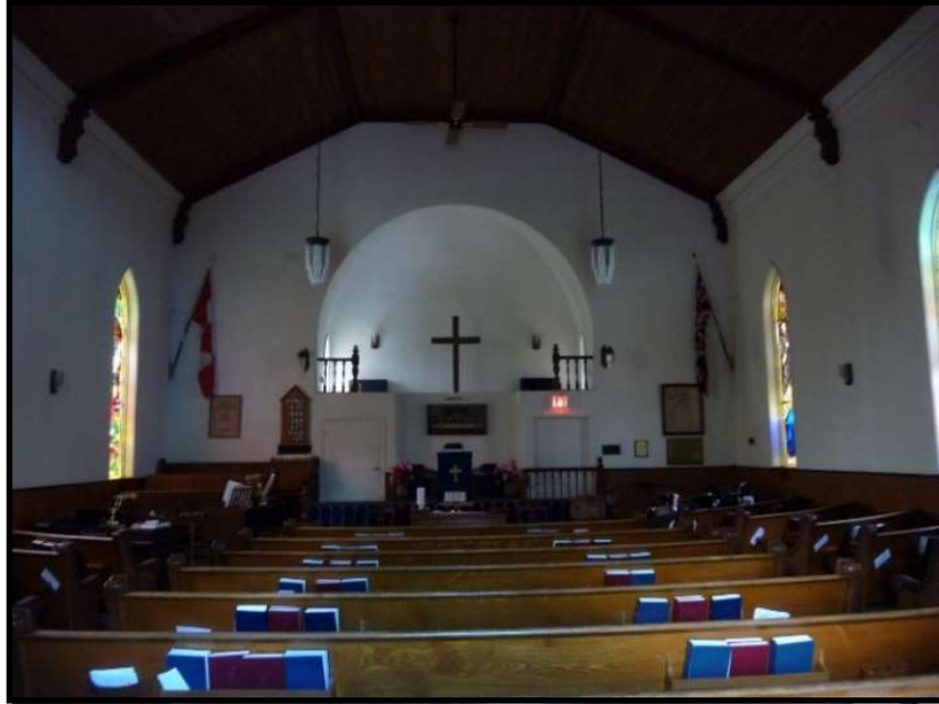
Figure 29: Nave showing the single-span, modified vault ceiling, September 2016
