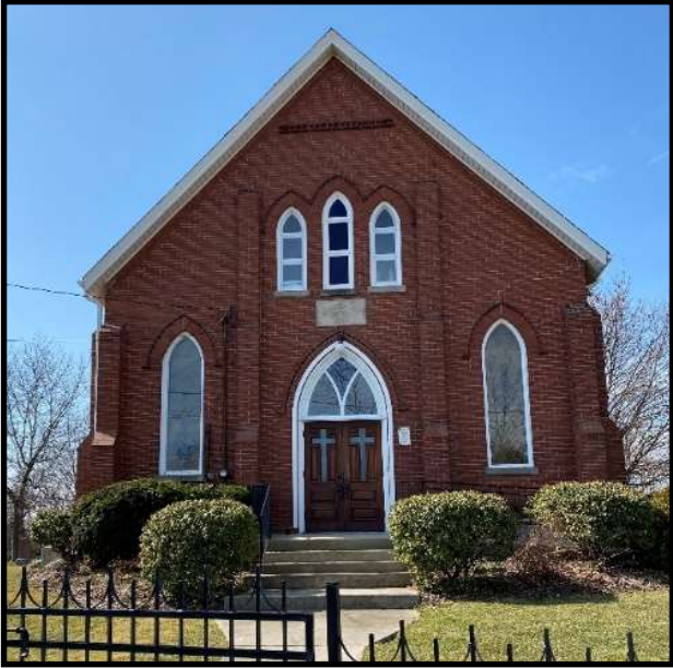
Figure 18: Front (east) façade, March 2020
