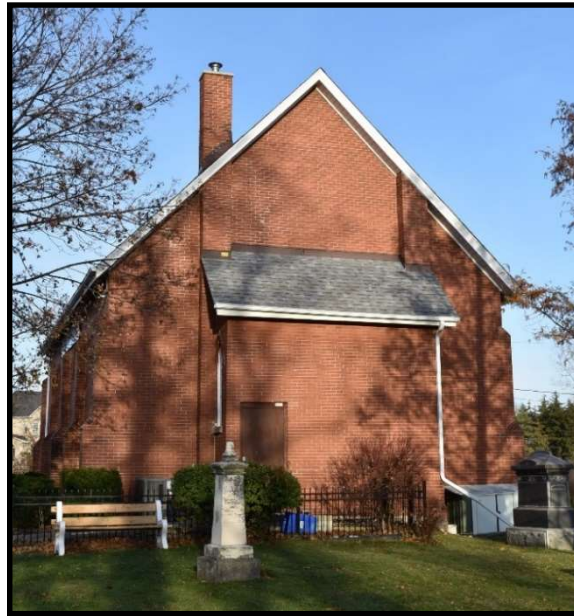
Figure 26: West elevation, November 2019
