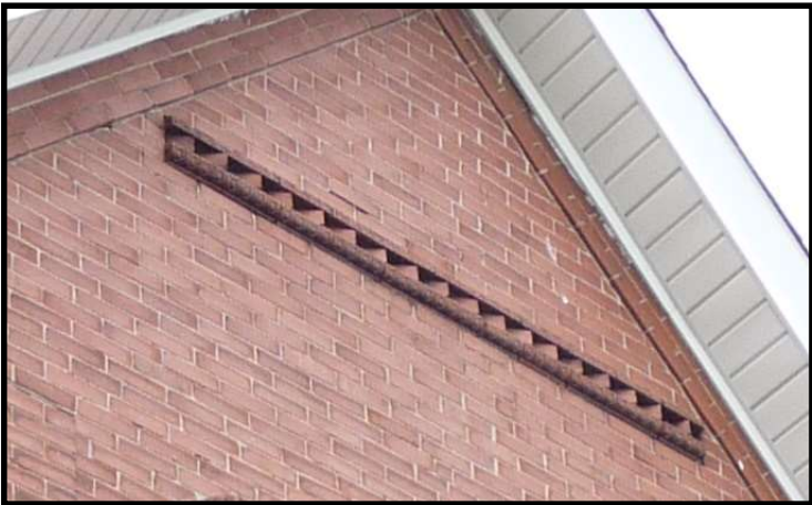
Figure 21: projecting dog-tooth course detail, September 2016
