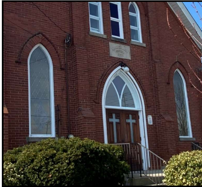
Figure 22: Front entryway buttresses and arched window details, March 2020
