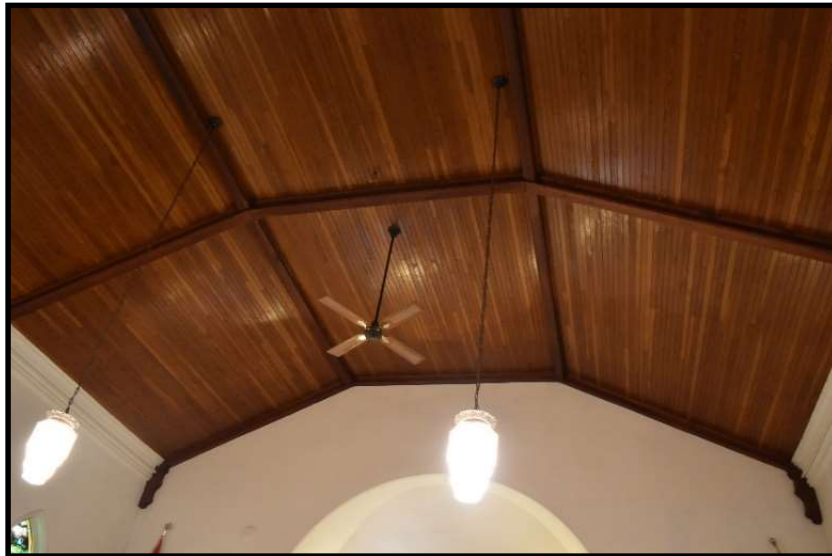
Figure 30: Nave ceiling, August 2019
