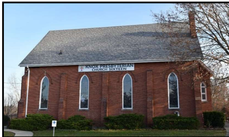
Figure 23: North elevation, November 2019
