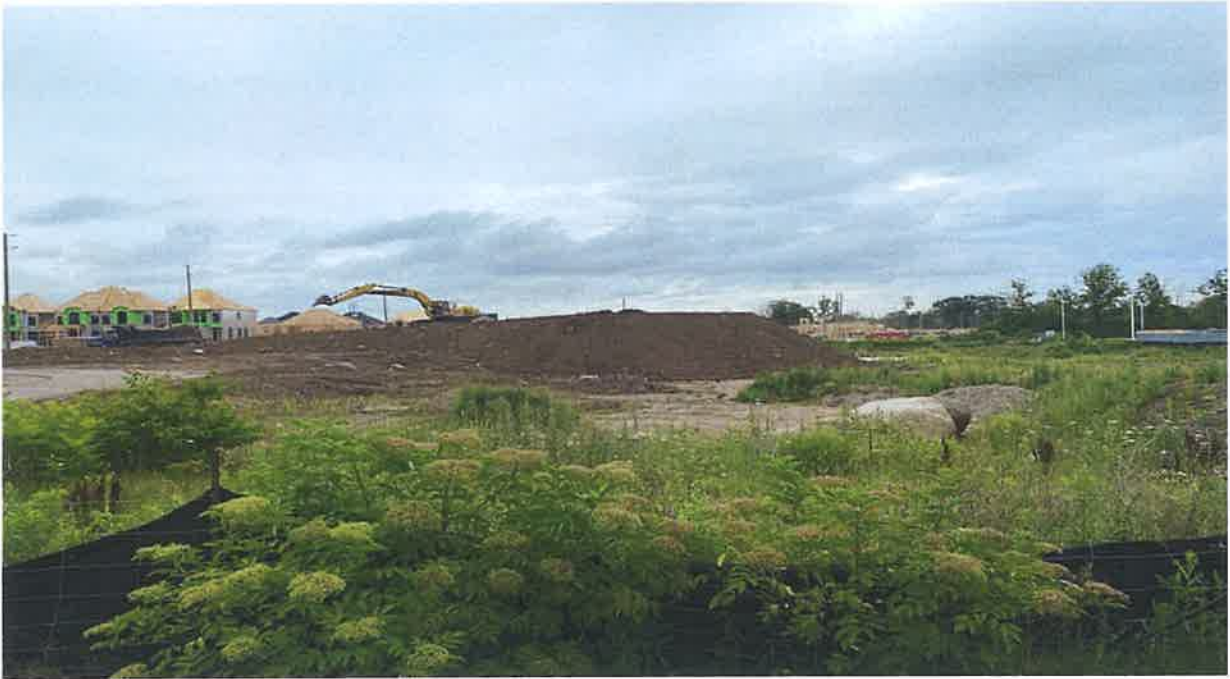
General view of subject site (looking northeast)
