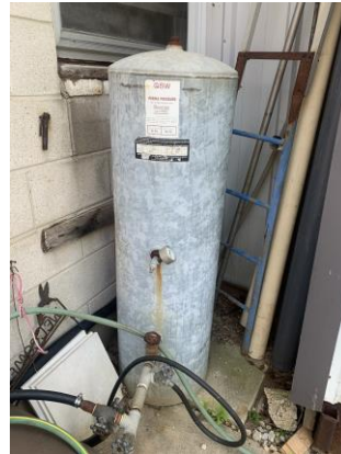
Picture 8: The pressurized water tank (used for irrigation of the garden) near the work shed.
