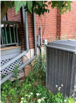
Picture 9: View of the vent pipes for the AST located at the basement of 1326 Bronte Road.
