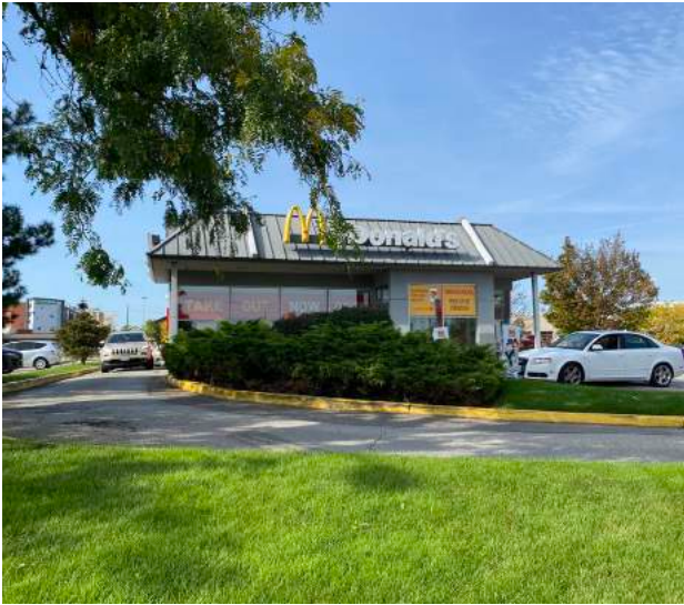
1 227 Cross Avenue, looking north.
