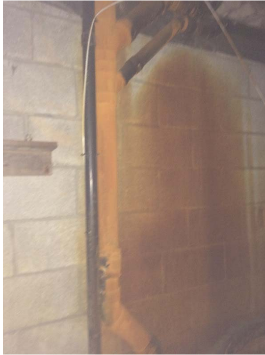
Photograph 13: Looking south, rust stains along southeast wall of house.
