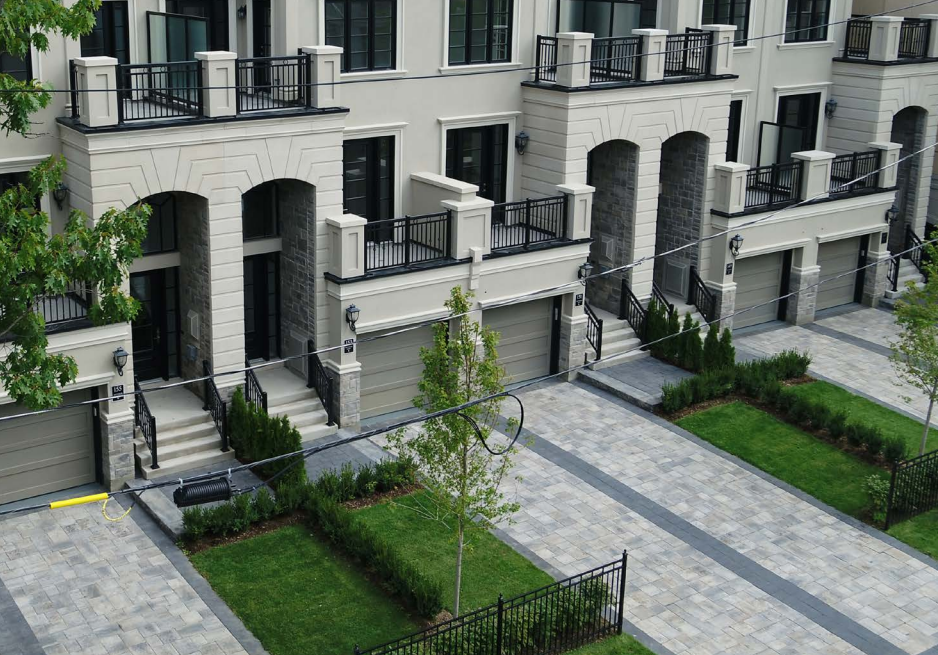
Figure 7.14: Landscaping example from 157 Reynolds Street Townhouse development.
