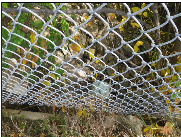
Ditch feature #3: Overlooking crossing structure and channel characteristics south of North Service Road East (October 8, 2013).
