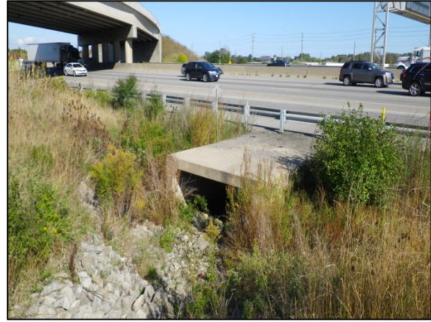
Ditch feature #2: Looking south (downstream) from upstream of the QEW (October 8, 2013).
