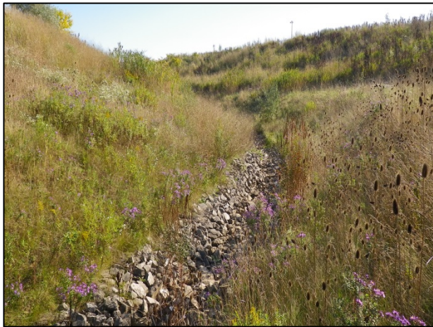
Ditch feature #2: Looking south (downstream) from downstream of North Service Road East (October 8, 2013).
